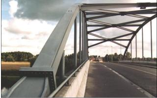
In 1990 ZINGA has been applied on the bridge of Melle (over the river SCHELDE). The whole bridge was first sandblasted. Then the complete structure was coated with ZINGA at 60  $\mu$ m DFT.
